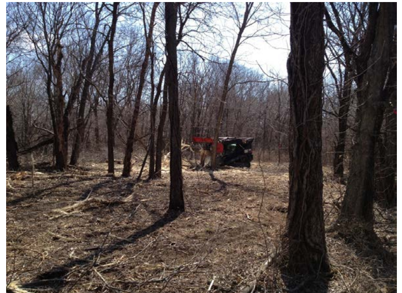
Clearing of Deer Creek Site Using a Tree-Mulching Attachment on a Rubber-Tread Skid Steer, Monitored by an Archaeologist
